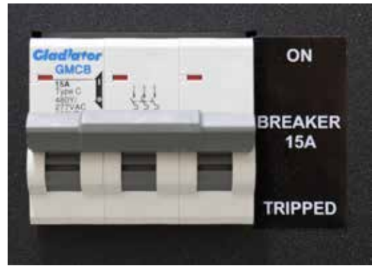
Figure 2.6 – AC Breakers
